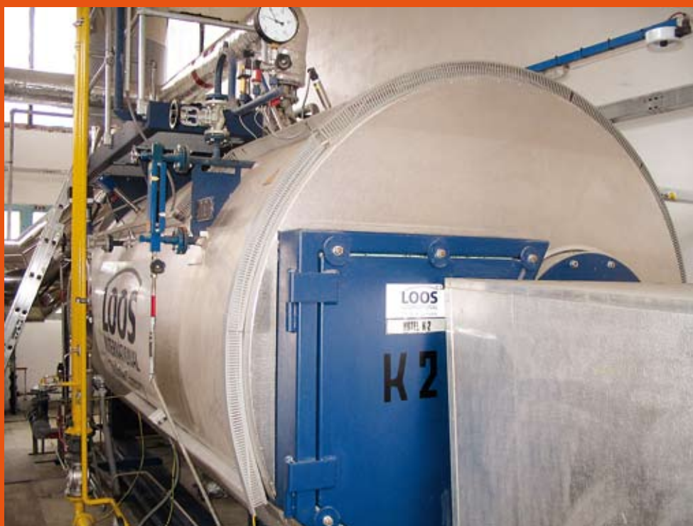
CNM Oskava - kotelna po rekonstrukci CNM Oskava - boiler house after reconstruction
