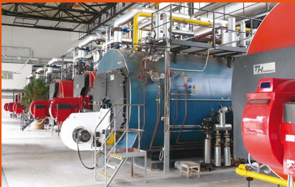
FN Brno - kotelna po rekonstrukci FH Brno - boiler house after reconstruction
