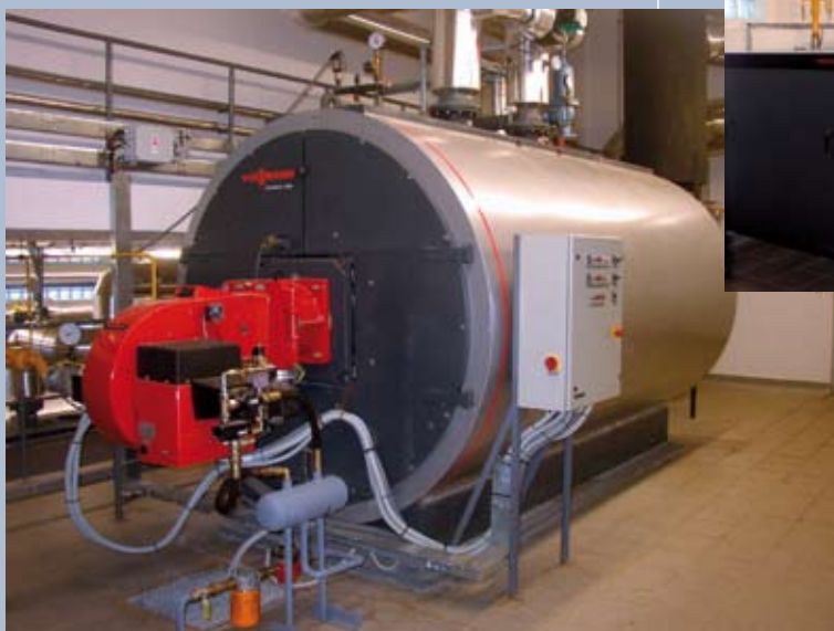
Technologie kotelny, Vimperk Boilers new situation, Vimperk
