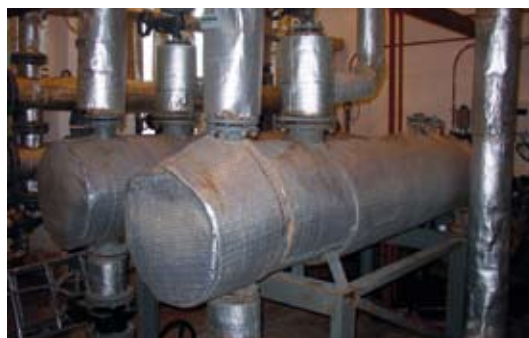
SPŠ Strakonice Secondary School of Industry in Strakonice
